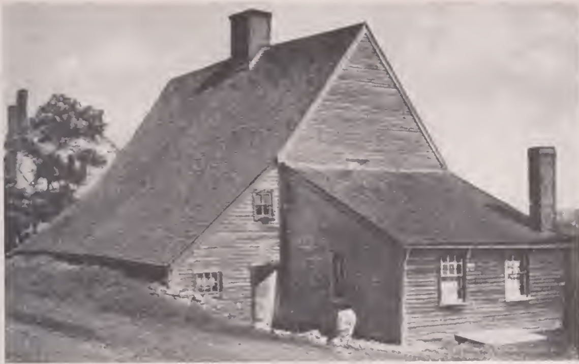
The old Jackson house, built in 1664, and probably the oldest now standing in Portsmouth, New Hampshire.
